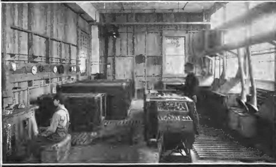
Dipping Room. Where the Float Bowls and Other Castings are Finished by Dipping After They Pass From the Sand Blast Department
